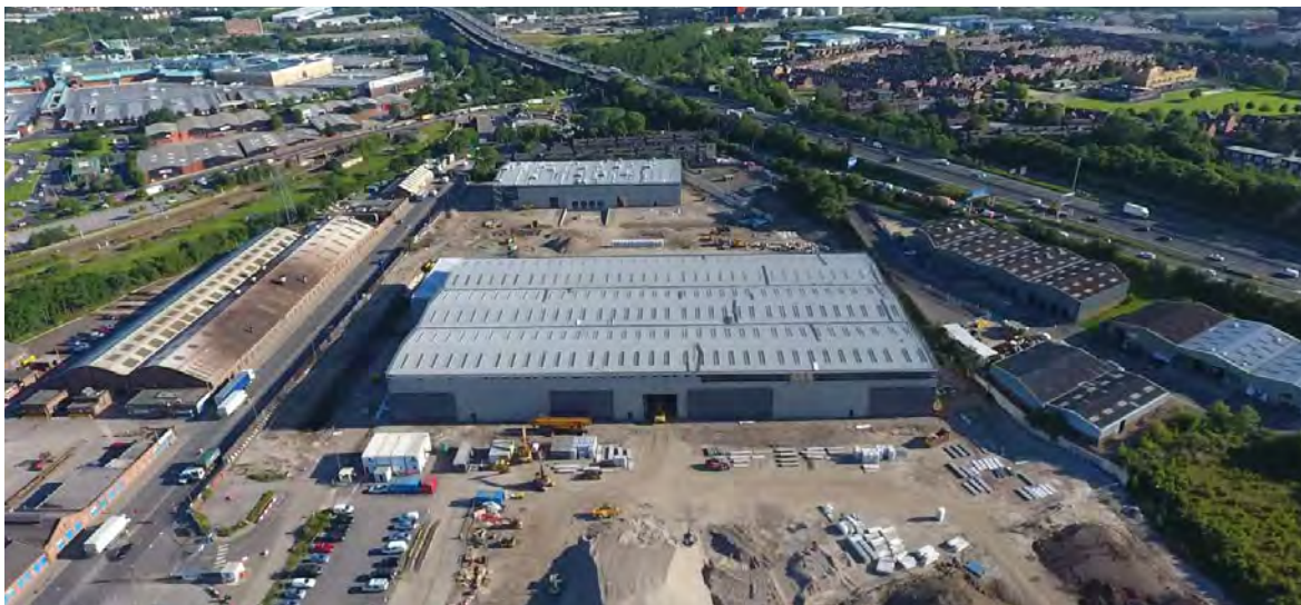
FIGURE 3.5 Electrolyzer gigafactory under construction in Sheffield, United Kingdom
