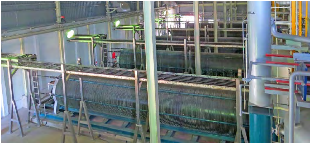
FIGURE 2.4 World's largest current electrolyzer (25 MW), polysilicon plant, Sarawak, Malaysia
