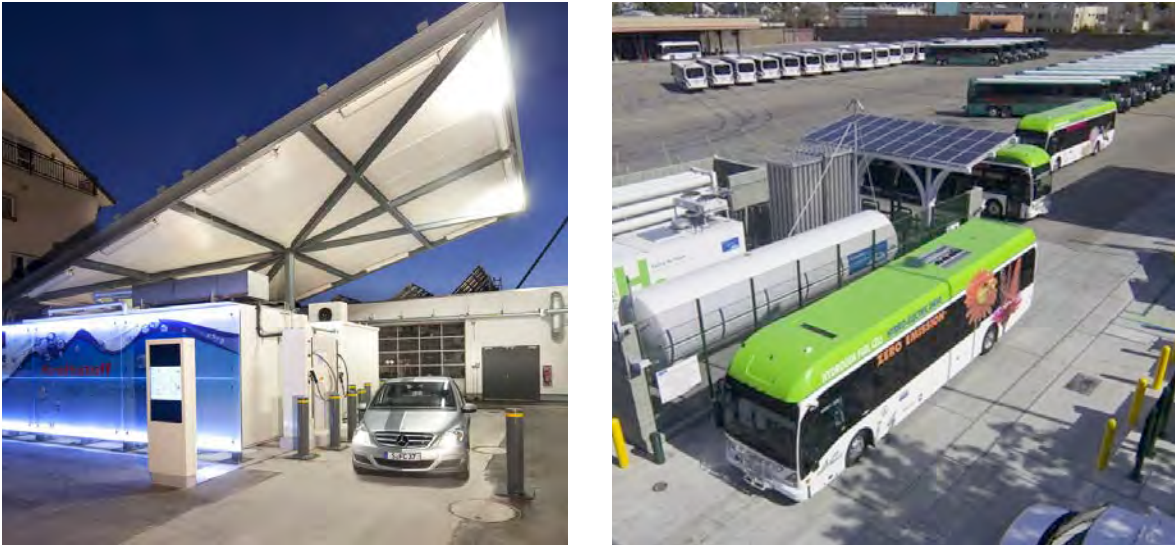
FIGURE 5.6 Green hydrogen refueling, with on-site hydrogen generation from rooftop photovoltaic: Freiburg, Germany, in 2012 (left) and Emeryville, California, in 2011 (right)
