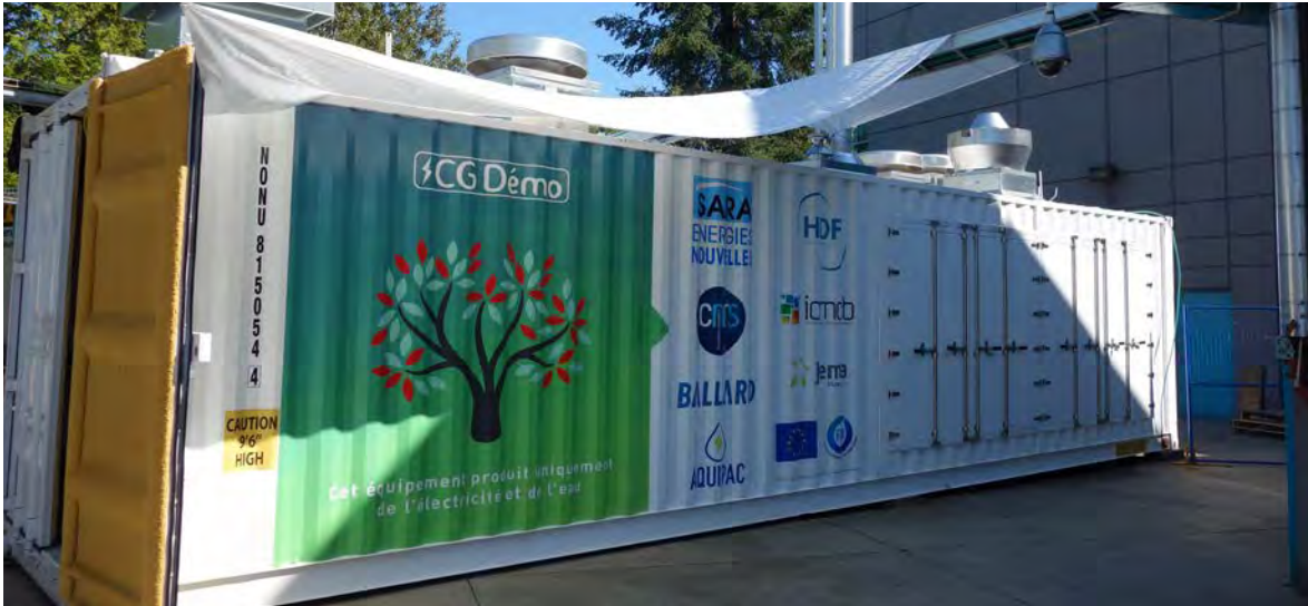
FIGURE 4.6 PEM fuel cell 1 MW unit using excess hydrogen from island refinery, Martinique, 2019
